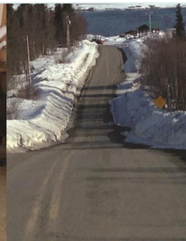
Aleknagik – Dillingham Road in winter
