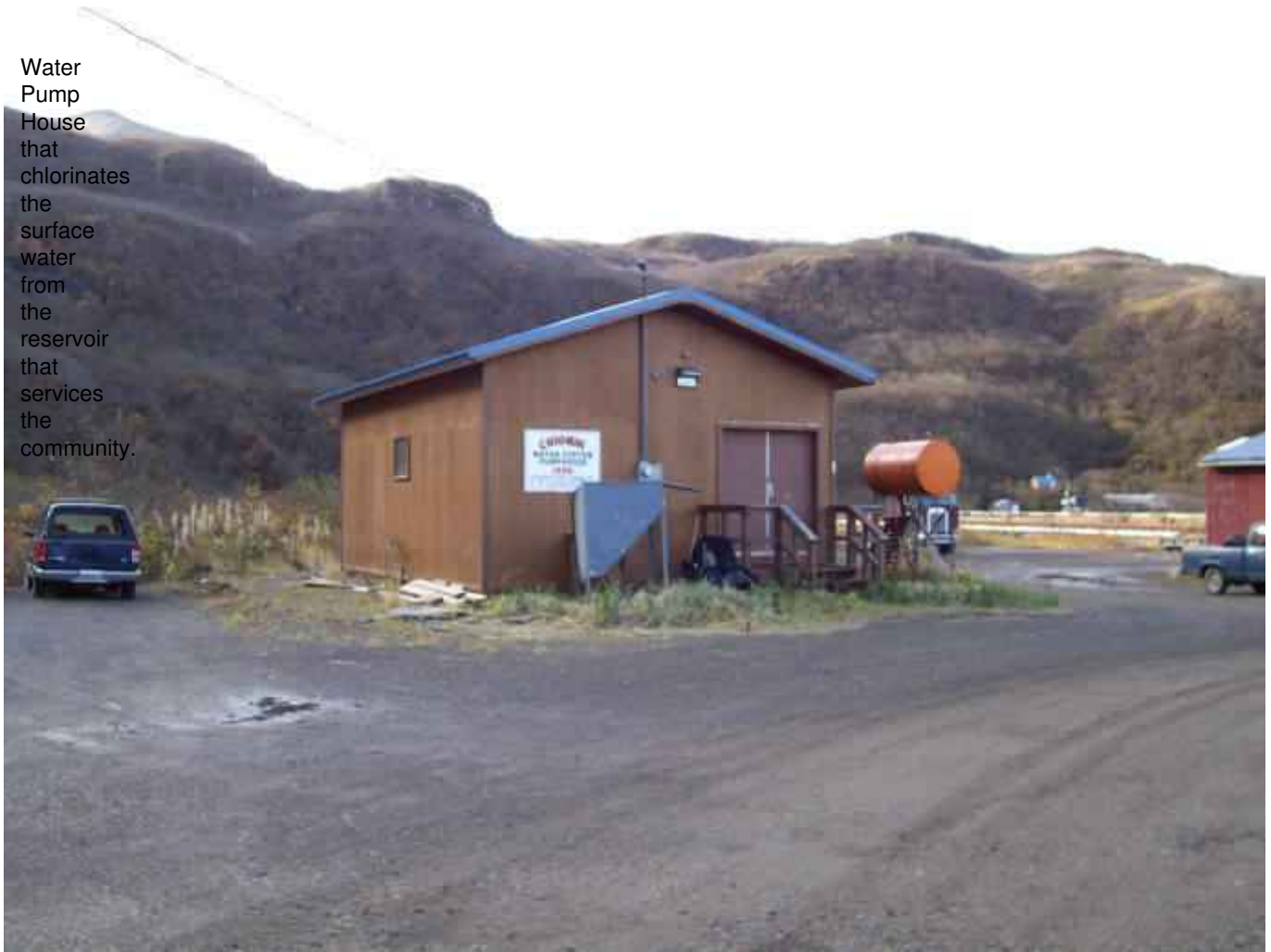
Water Treatment Plant Building: East Side
