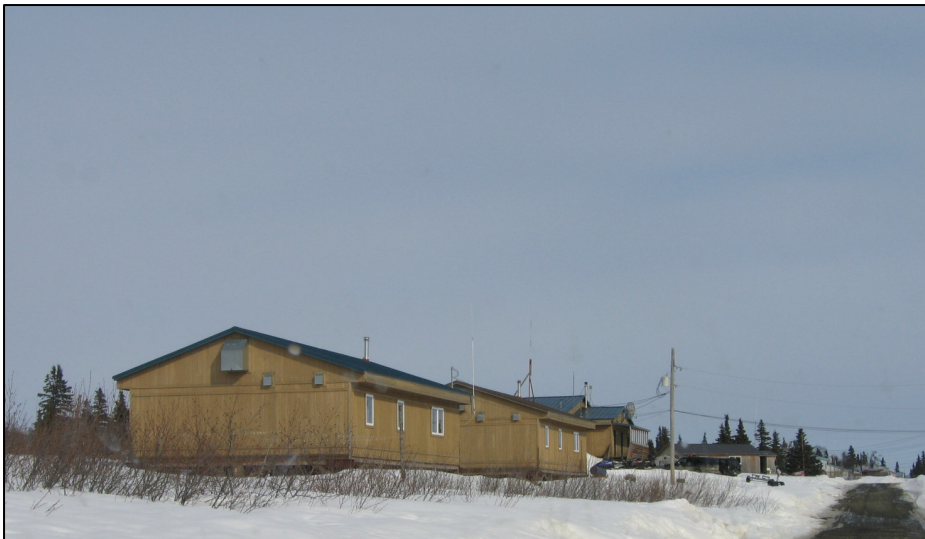
Housing at Manokotak Heights
