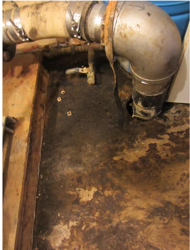
Figure 11: Deteriorating floor in booster station.
