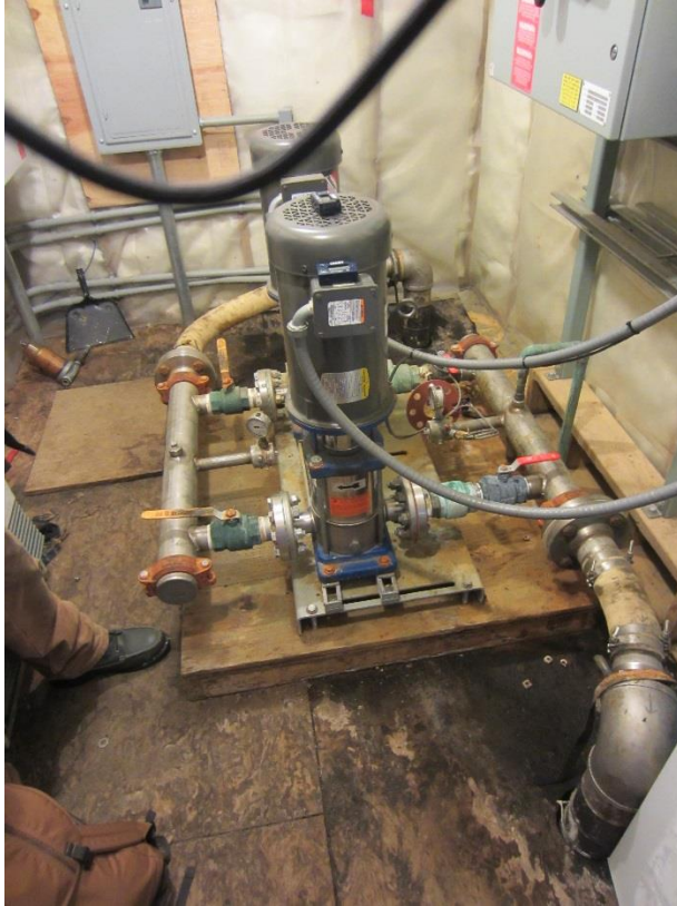
Figure 11: Deteriorating floor in booster station.
