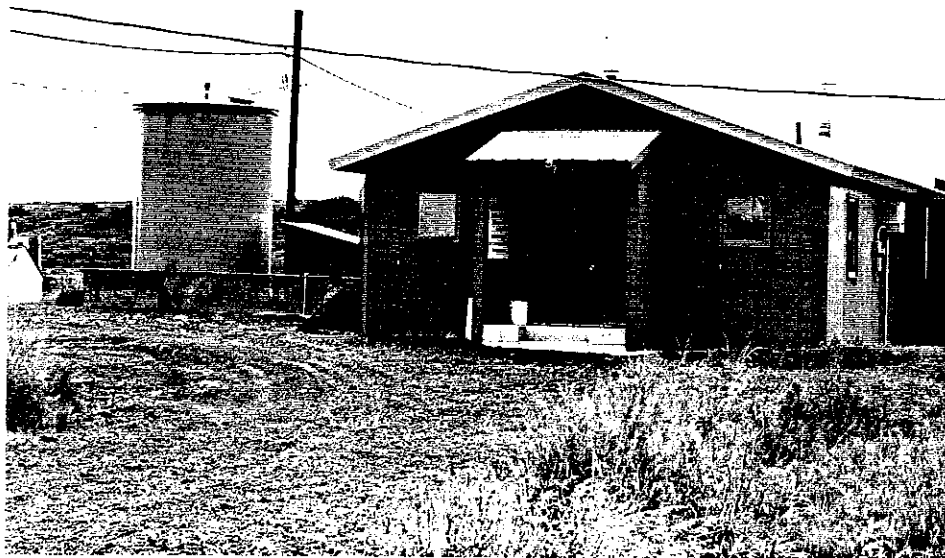
Twin Hills Pumphouse (courtesy of DOWL Engineers)
