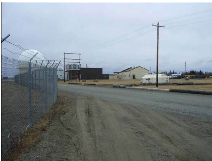
King Salmon AFS bulk fuel storage area, emergency power generation and satellite communications. Photo by Vivian Melde, May 2010.
