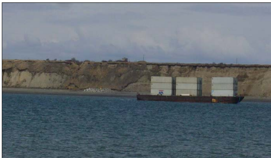
Erosion impacts on the bluffs of the Naknek River, below the Borough sewage lagoons. The pump station for the sewage line is near the middle of the photo, taken from South Naknek by Vivian Melde, May 2010.
