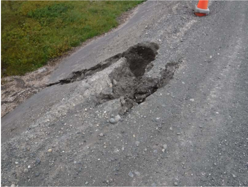
Photo 11 - Roadway erosion
