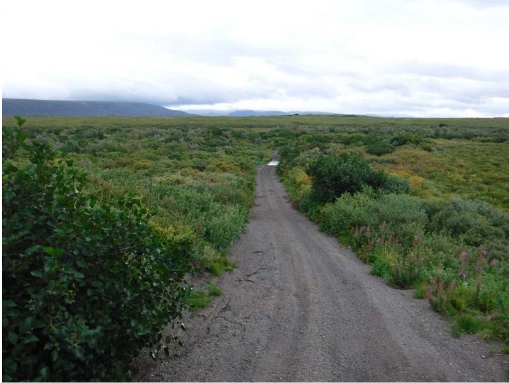
Photo 07 - Stream crossing ATV trail with no bridge
