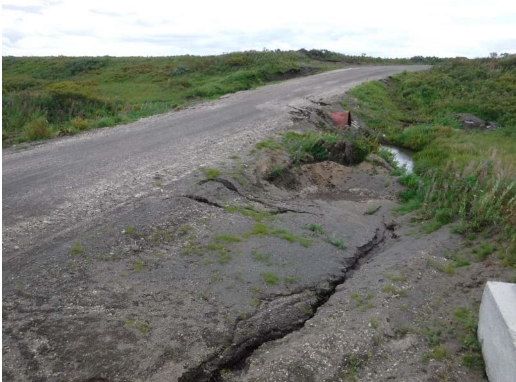
Photo 08 - Eroding shoulder
