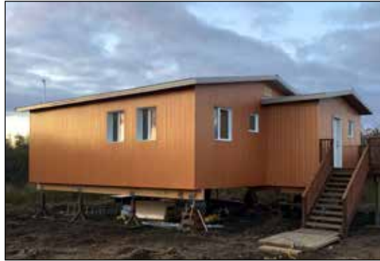
New standards for construction, Ulroan Home.
