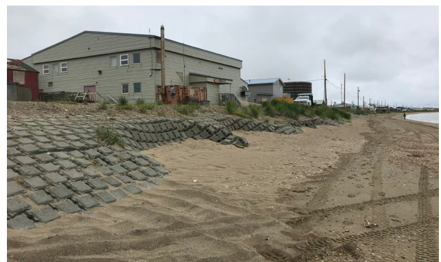
Figure 12. Erosion control structure at Deering, which was undermined and damaged by storm surges. Photo taken July 2018.
