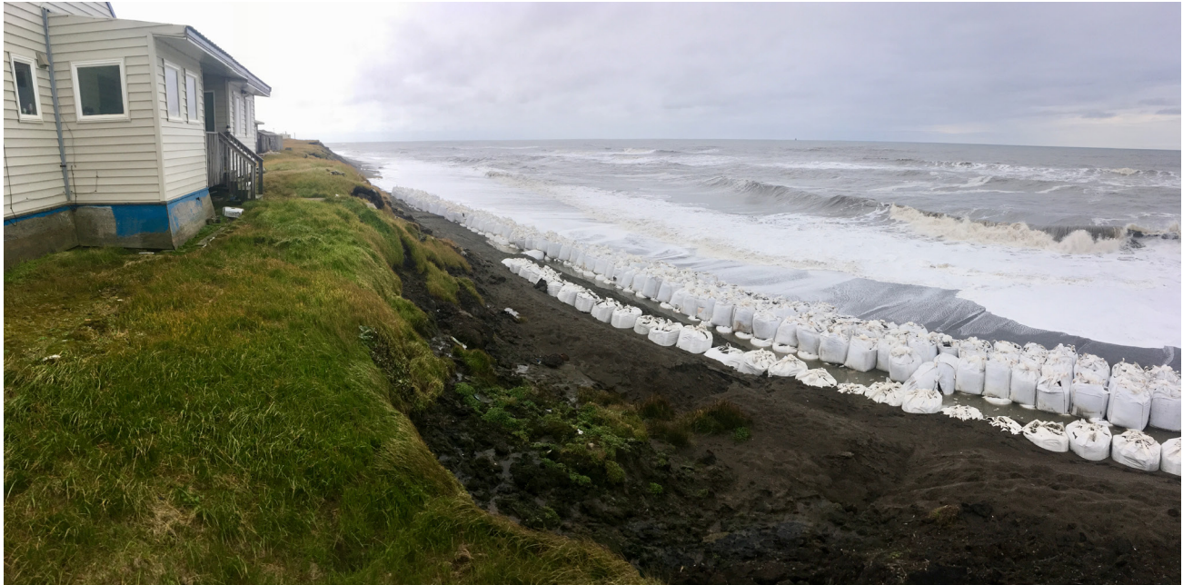
Figure 6. Erosion of ice-rich coastal bluffs at Utqiagvik during a coastal storm. Photo taken August 2019. Sandbags have been placed at the base of the coastal bluff to mitigate erosion.
