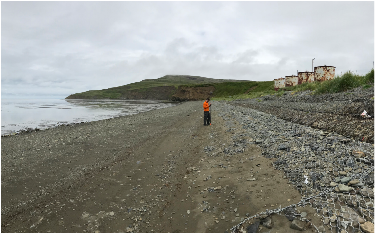
Figure 19. Gabion basket revetment at Tununak, August 2019.
