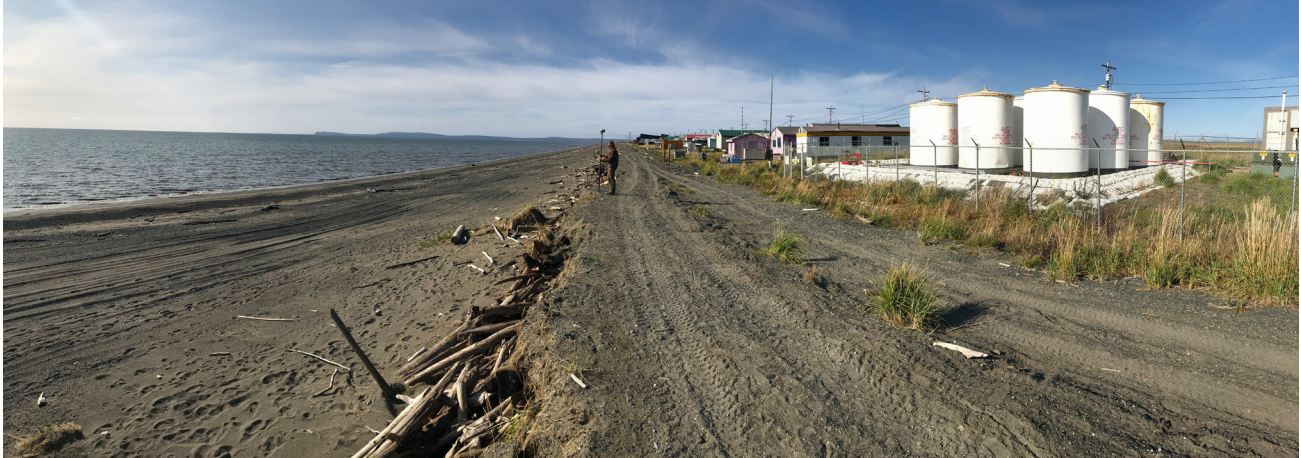
Figure 13. Unconsolidated gravel berm (used as a road) in front of the tank farm in Shaktoolik. Photo taken after a storm in August 2019 eroded the berm.
