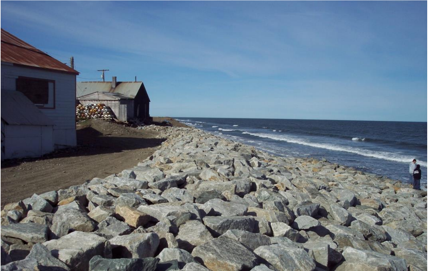
Rock revetment at Shishmaref, Alaska. Photo: Orson Smith, PE, Ph.D., University of Alaska Anchorage
