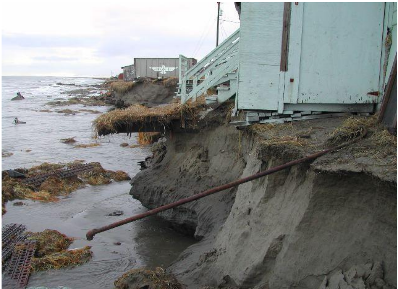
Teacher housing threatened by erosion in Shishmaref. Photo: Kawerak
