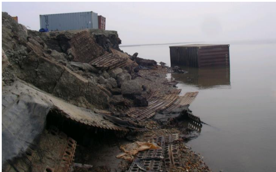
Newtok barge landing, erosion damage. Photo: Department of Commerce, Community, and Economic Development, Division of Community and Regional Affairs (DCCED/DCRA)
