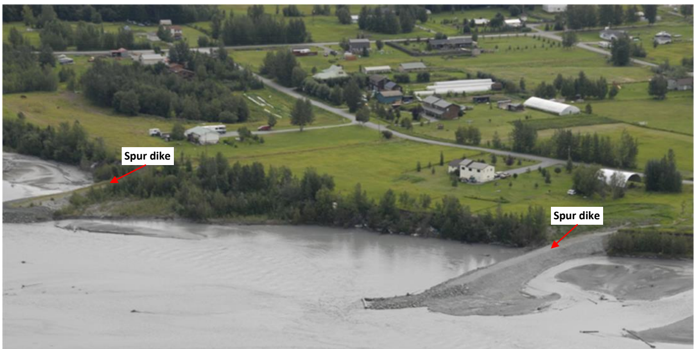
Spur dikes on the Matanuska River. Photos: U.S. Geological Survey (USGS)
